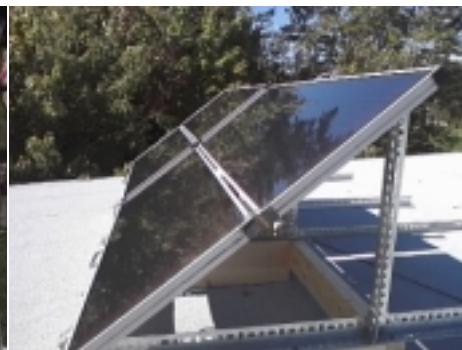
Panels mounted to steel frame and wooden base
