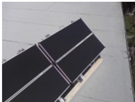
Panels mounted to steel frame and wooden base
