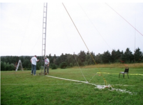
With the tower standing, the derrick and its rigging lie on the ground
