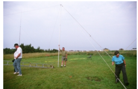
The tower lies down while AI steadies the derrick and Helen checks guys & stakes
