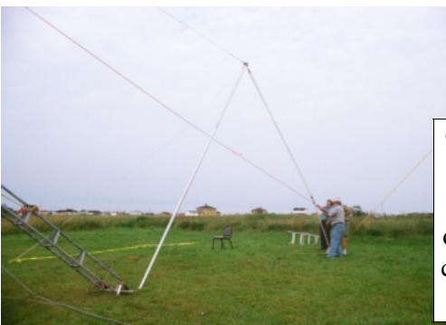
Tower going up; derrick coming down
