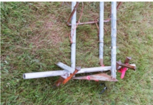
The base is firmly staked to the ground and the bottom of the tower rotates around the piece of pipe
